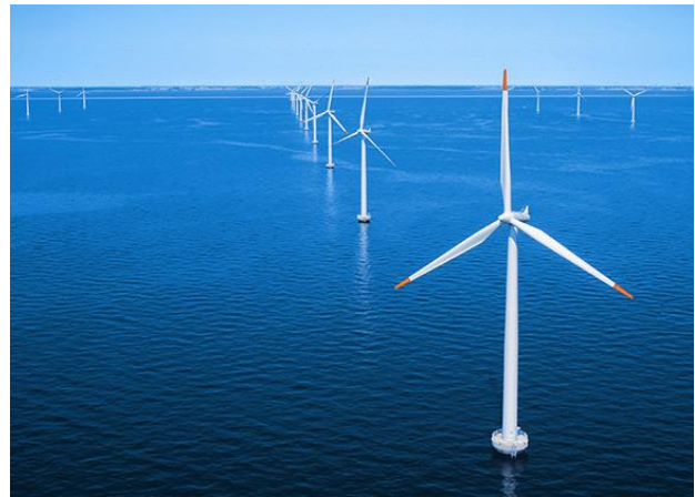
Exhibit 11: Off-shore wind turbines
